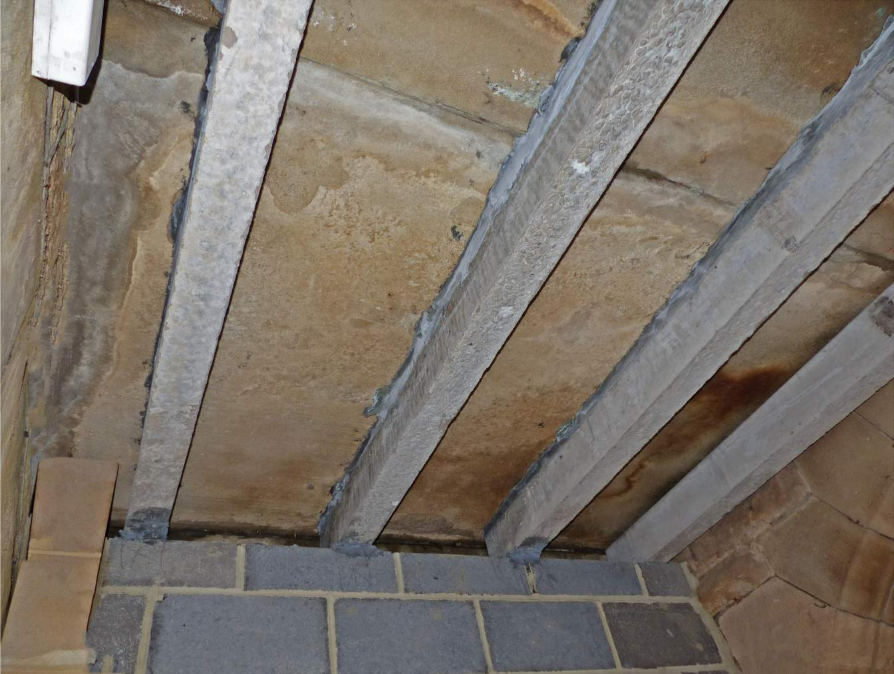
Concrete lintels inserted into retaining wall brickwork
